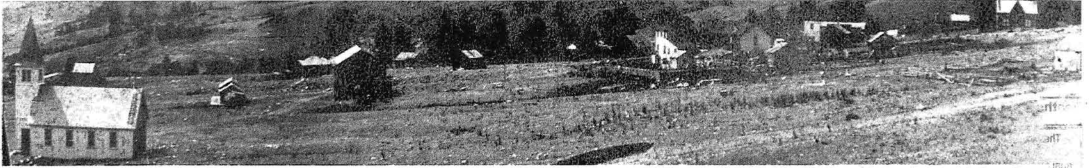
The Blasted Church, shown in about 1900 at its original location at Fairview town site gold mine, was blown up and reconstructed at Okanagan Falls and is now featured by a local winery. Story, C3.
